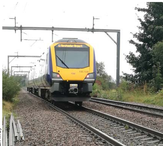
Train crossing Chat Moss—as trains pass, the ground gently quakes, presumably on its original 1830s brushwood mats and foundations
